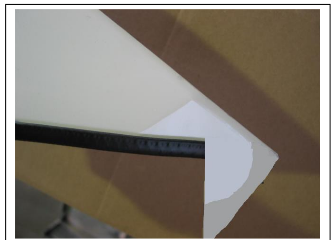
Figure 8: 3mm clip lock, trimmed to suit rear of cut off
